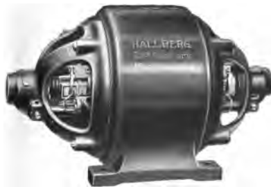
Hallberg Motor Generator 60 cycles A. C. to D. C.
